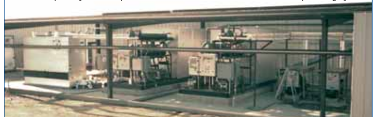
Two 43 ton per day modular plate icemakers for broccoli and sweet corn liquid icing system
